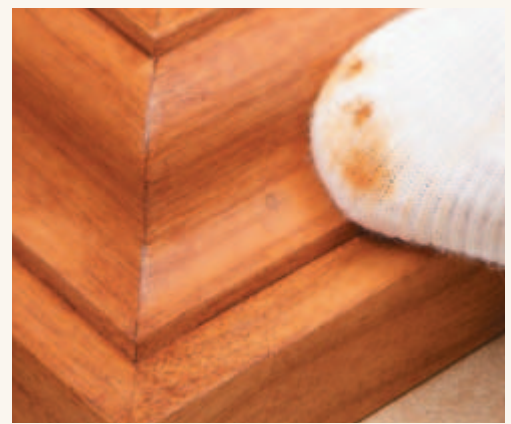
▲ Wipe Away Excess. With a soft cloth remove the excess putty and buff away any residue from the surrounding surface.
