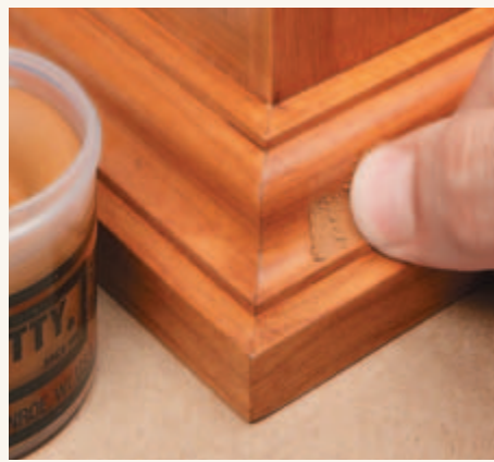
▲ Apply the Putty. Press a small dab of putty over the nail hole. Work it in so the hole is completely filled.
