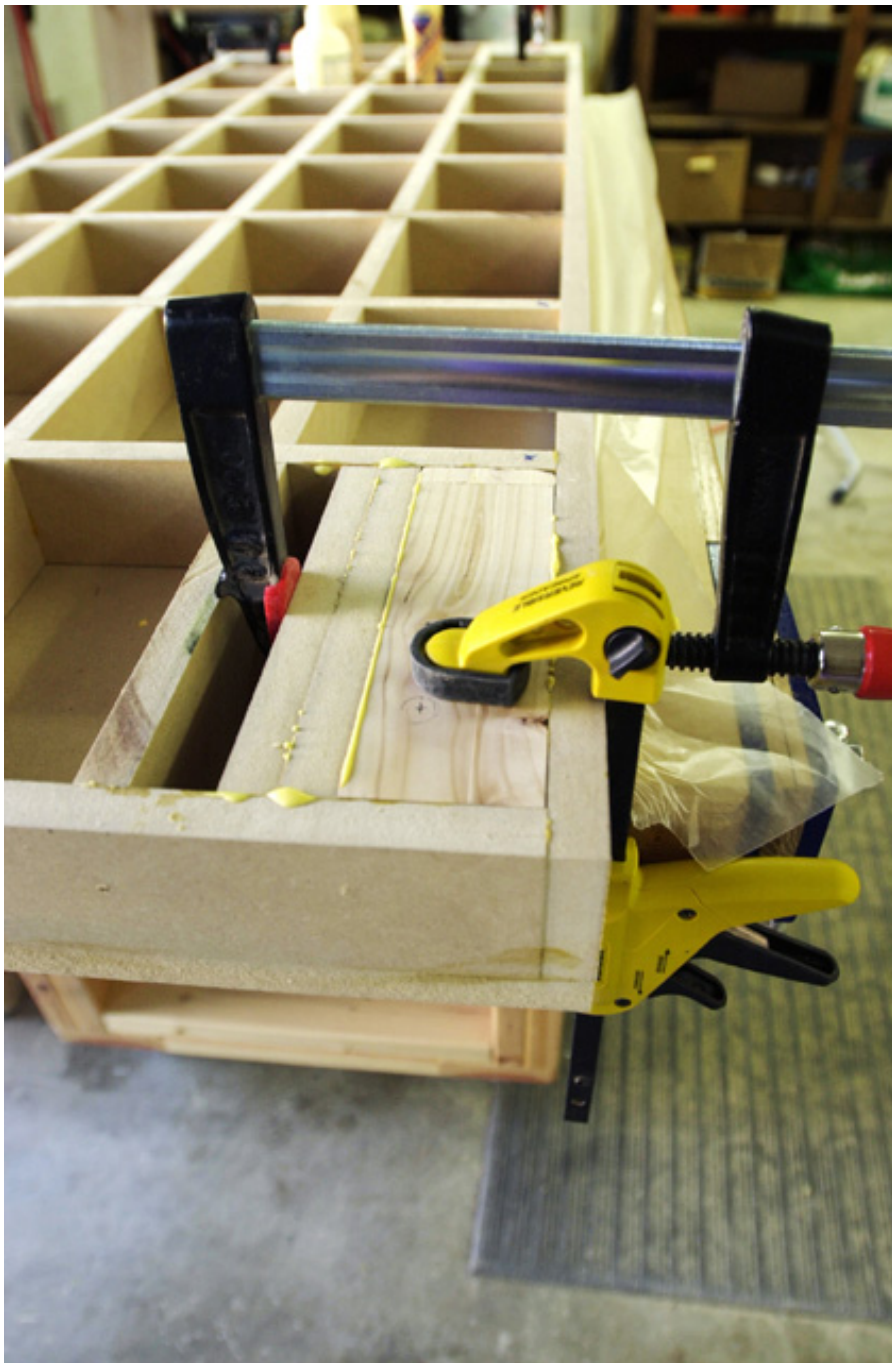
Hardwood fillers in the corners provide some meat for the casters to lag into.
